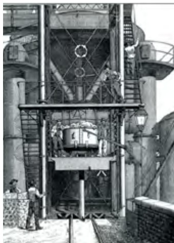
Fig. 47. Details of Bell for Closing Mouth of Furnace.
