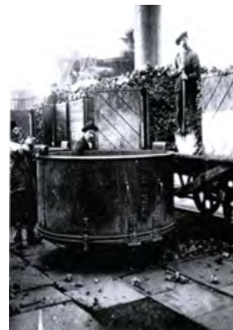
Fig. 47. Details of Bell for Closing Mouth of Furnace.
